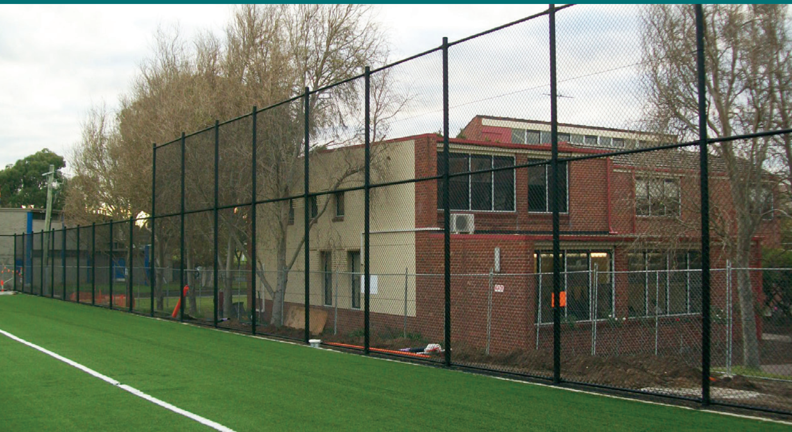
High screen chain link fence with black powder coating at Brighton Grammar. Photo: Lee Brothers Group Fencing
