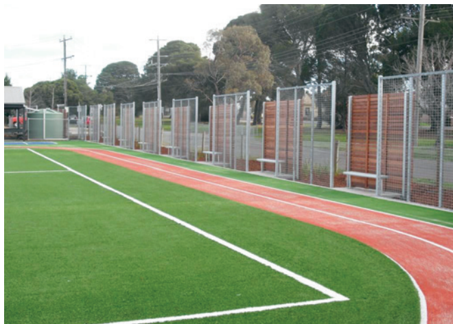
Custom timber panels with galvanised tubular steel and weld mesh. Photo: Lee Brothers Group Fencing
