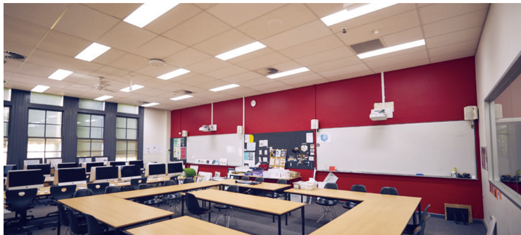
Using a combination of LED tubes, globes and exterior floodlights, Westall Primary has improved lighting quality in the school, and saved 65 percent on their lighting energy consumption. Photo: Shine On
